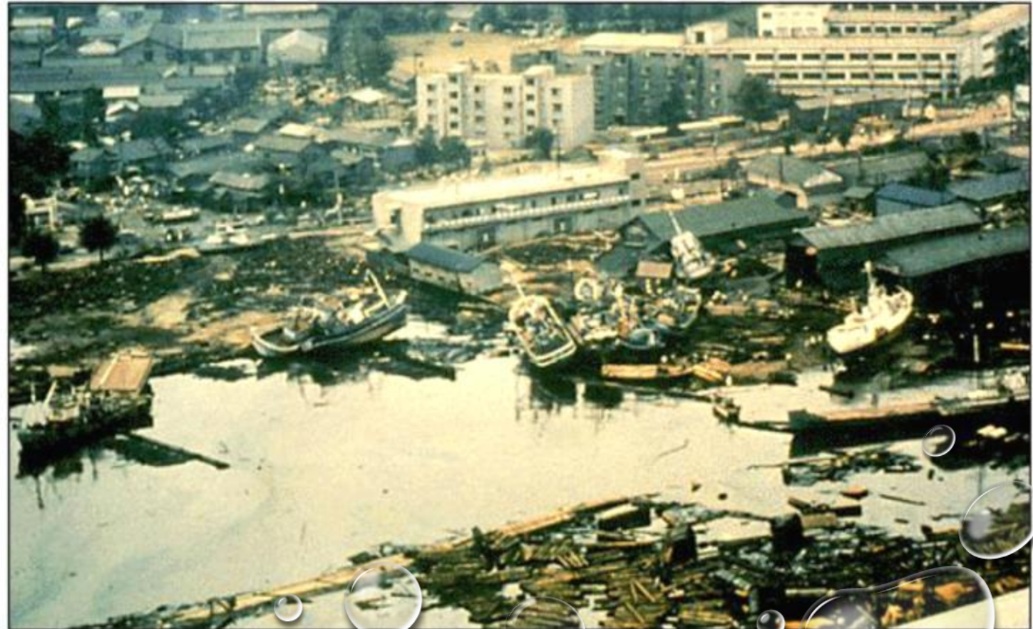
Destruction caused by a tsunami in Niigata, Japan.
