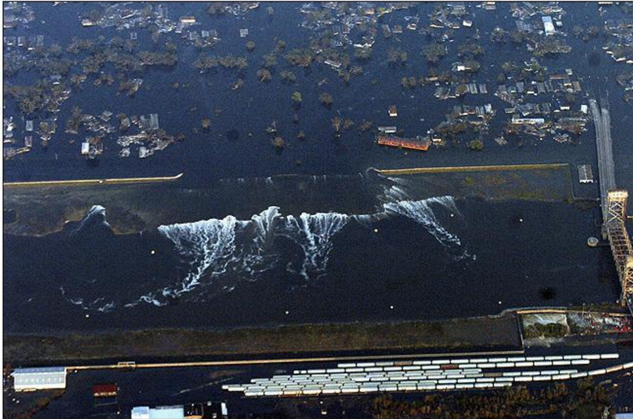
Caption: breached levee.
